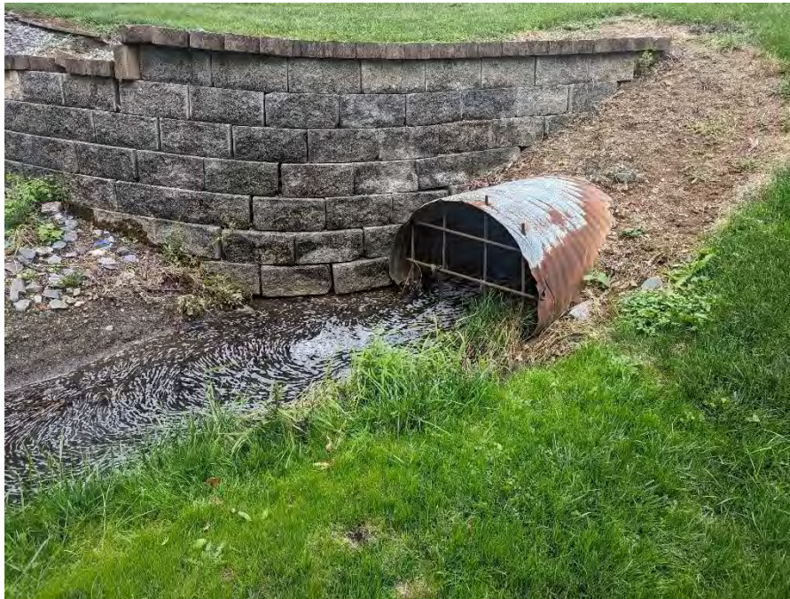
Photo 1: Image of outfall. Water ponding at location in slight pool.
