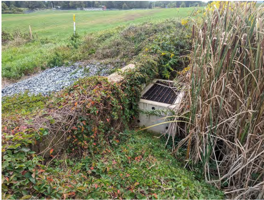
Photo 3: Outlet structure. No clogging from vegetation.
